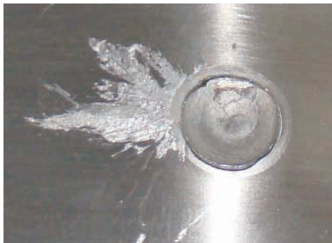
Fig. 7. Metal spurt between welded aluminium alloy sheets
